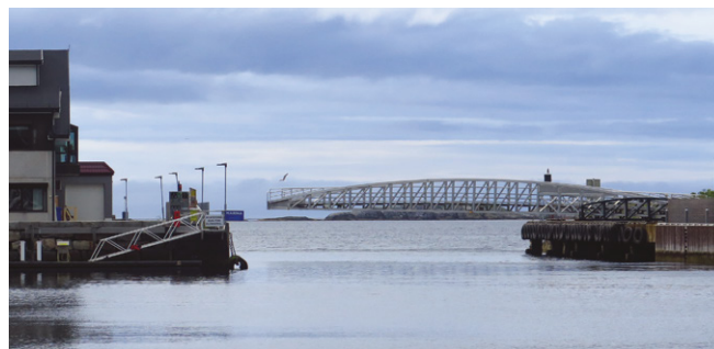
Pedestrian swing bridge, Fosnavåg John Sadd
