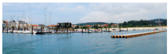
The new (2017) breakwater at Porto Novo Geraldine Hennigan
