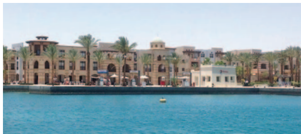
Port Ghalib international marina bunker station fuelling berth
